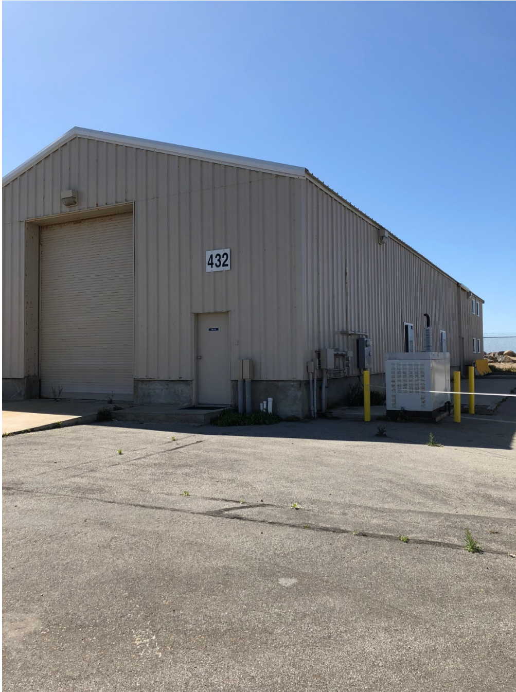
Photo 1. Building 432 Two story warehouse building - approximately 4,446 sq feet
